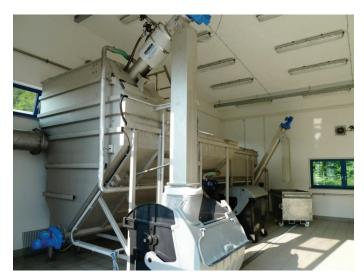
Complete Plant the building volume for the required mechanical equipment and thus the building costs could significantly be reduced. In the mid term, the options integrated in the Complete Plant – screenings washing and grit trap material washing – will pay off because they considerably reduce the volume of waste which requires disposal.
