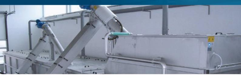
The Pemberton WWTP was recently upgraded to increase capacity and discharge quality. Part of the upgrade included a HUBER Ro5 Packaged Inlet Works.
