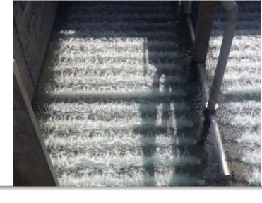
"The main benefits of the AEROSTRIP® diffusers are the significant power savings they achieve by the high oxygen transfer rate 4.0-5.0 kgO2/kW and the robustness of the membrane, which has a proven life of greater than 12 years.
