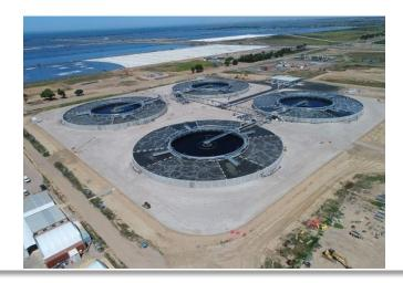
Melbourne Water's Western Treatment Plant (WTP) has been recently been upgraded to include a new 140 ML/d process train.
