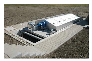
The removed solids are washed into a trough situated below the segment openings prior to being discharged and the filtration process runs on continuously whilst the filter discs are being cleaned. The resulting level difference between the water level inside the central shaft and inside the concrete tank is the driving force within the filtration process and renders unnecessary wastewater lifting or sucking off
