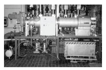
The total mixed sludge is screened immediately before the heat exchangers. The fibrous material and hair are separated from the sludge flow and compacted. 60 m<sup>3</sup>/ hour of mixed sludge are fed into the STRAINPRESS<sup>®</sup> by gravity or vacuum forced through the machine by pumps behind the coarse material separators. The inlet concentration of the primary sludge is between 2 and 3% DR.
