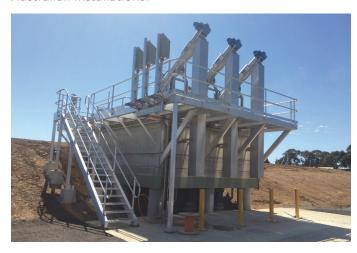
The screens are fully fabricated in 316SS and the drum is provided with 2mm perforations to remove very fine material, fibre, plastics and cotton bud sticks.
