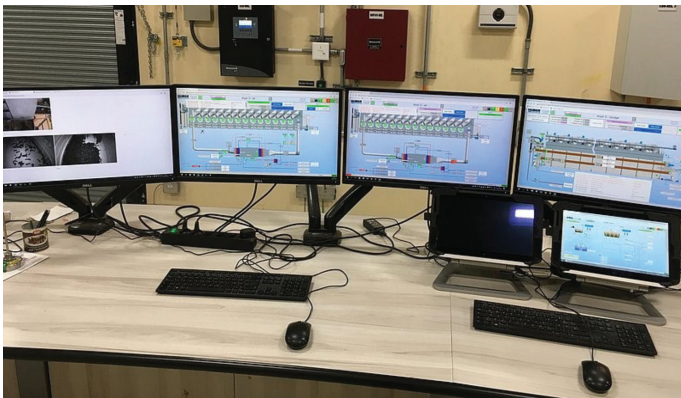
Control system for the drying plant
