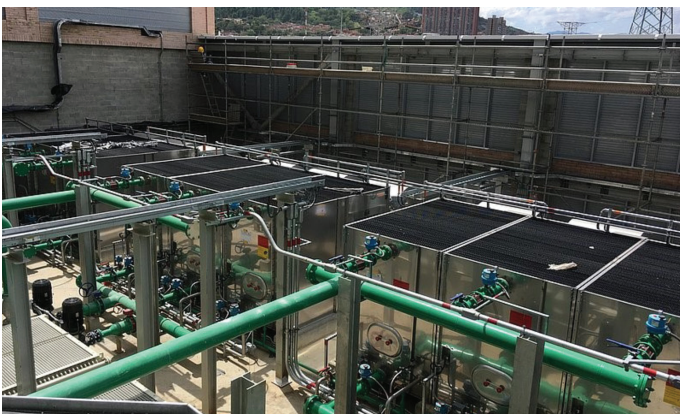
Cooling towers and exhaust air treatment
