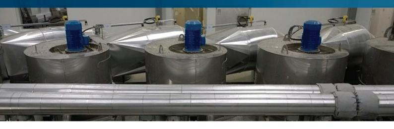
On the Isle of Man, up to 12,775 t sewage sludge per year will efficiently be dried from now on. HUBER received the order to build a belt dryer on the Isle of Man at the beginning of 2015. The customer wanted to reduce the energy expenditure for sludge drying and the resulting high disposal costs. The HUBER BT 16 achieves this most impressively.
