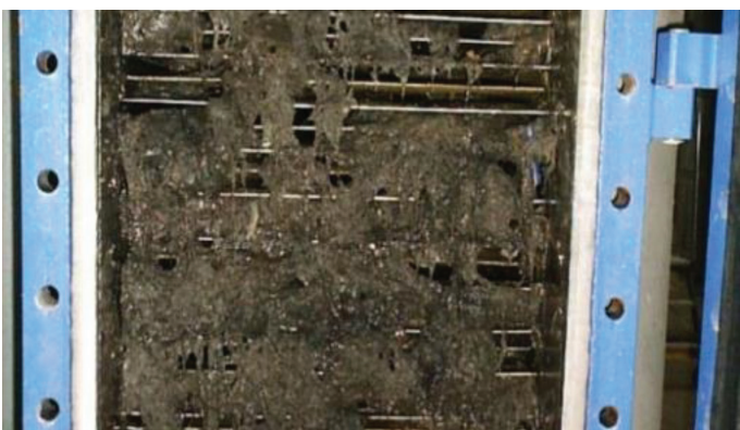
Blocked Heat Exchanger, reduced efficiency
