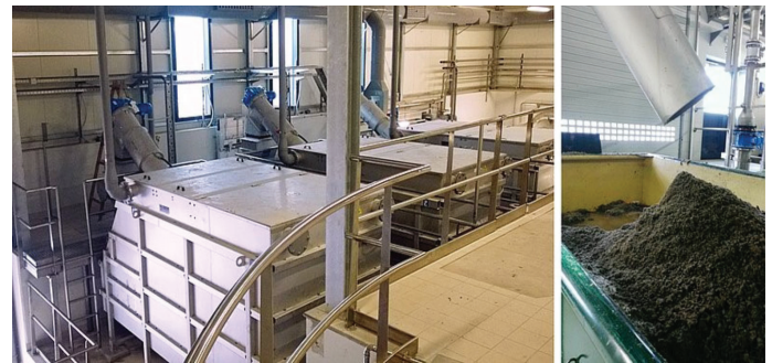
Fine Screen HUBER ROTAMAT® STAR with a throughput capacity of 1.000 m 3 /h each providing excellent dewatering results of > 35 % DR
