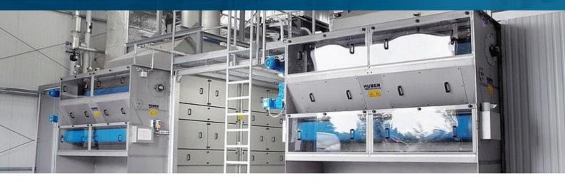
Two HUBER belt dryers type KULT BT 80 were put into operation on STP Ingolstadt in August 2005. The installed total dryer surface is 160 m<sup>2</sup> which is the same as that of our new dryer type BT 16.
