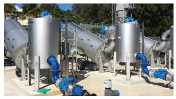
The technology installed is the HUBER Rotary Screw Thickener. This process uses an internal screw housed within a wedgewire drum.
