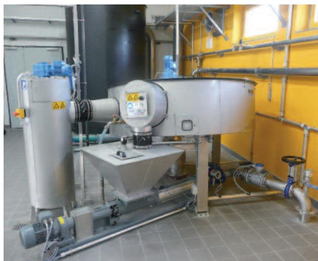
*ROTAMAT® Disc Thickener RoS 2S designed to thicken 35 m<sup>3</sup>/h*
