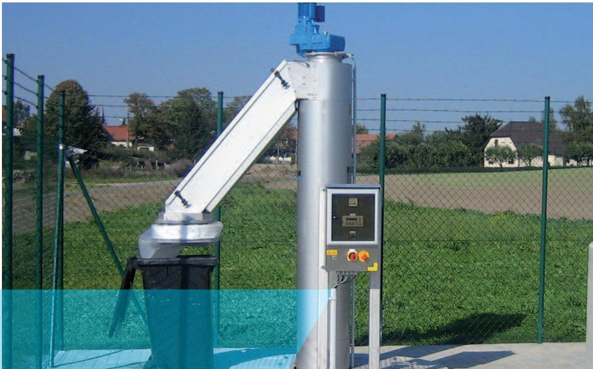
Automatically cleaned fine screen with vertical lifting, dewatering and compaction of screenings
