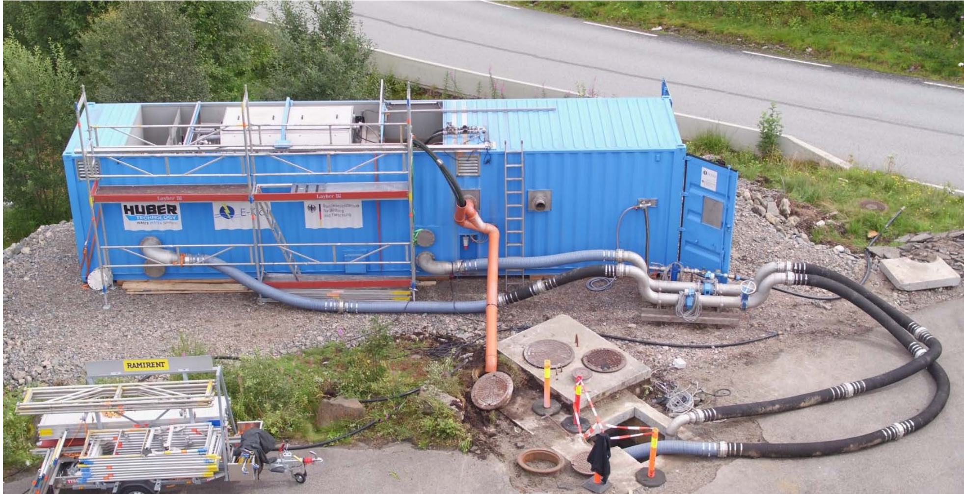
Full scale container plant 12m long x 3m wide x 3m tall (39'x10'x10')
