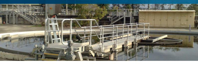
A Hydroflux Epco HeadMax Suction Tube Clarifier mechanism was installed into an existing clarifier at the Brendale STP.
