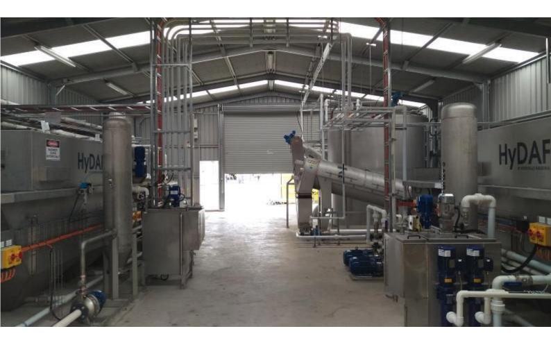
■ The Hydroflux HD-DAF system is specially designed for the treatment of municipal wastewater with proven systems successfully operating in numerous applications.
