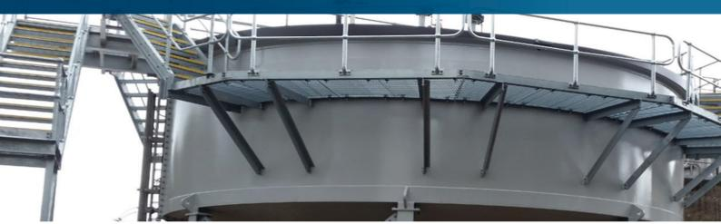
The Landers Shute WTP operated by SEQ Water was recently upgraded by Stirloch Constructions to include a new pre and post lime dosing system. A Hydroflux Epco Lime Saturator was included as part of the works.
