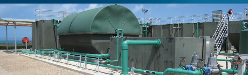
Based on successful Roadtrain<sup>®</sup> installations at Masig and Erub Is, a 100 m3/d system was installed at Mabuiag Island, located in the Torres Straits.
