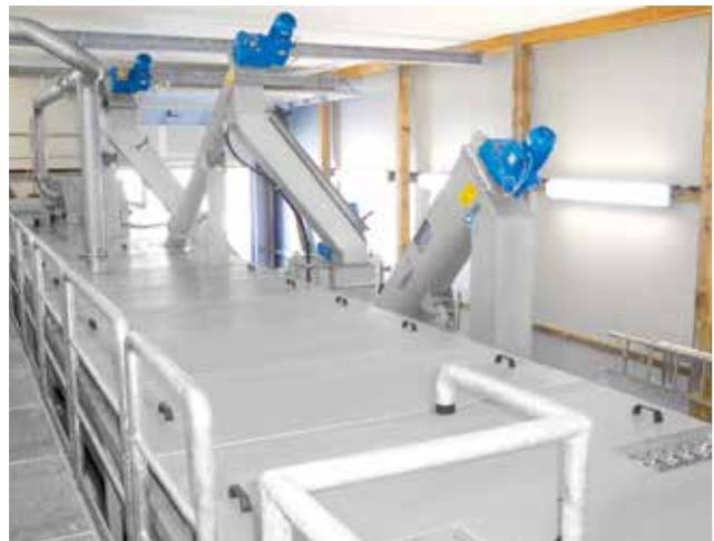
*Odour-encased screenings discharge from the HUBER Complete Plant ROTAMAT® Ro5.*
