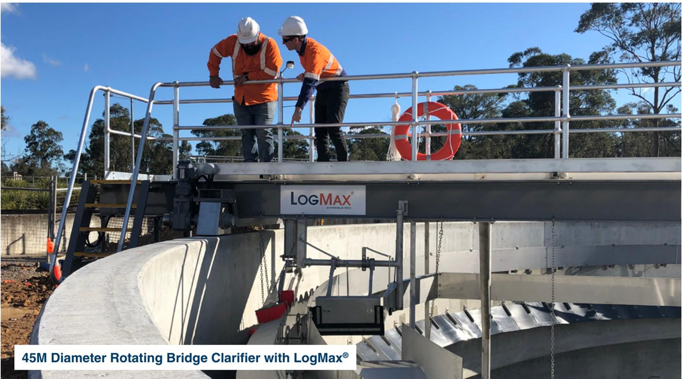
45M Diameter Rotating Bridge Clarifier with LogMax®
