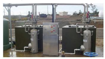
volatiles in the sludge, provides pathogen removal within the sludge and generates biogas which is rich in methane.
