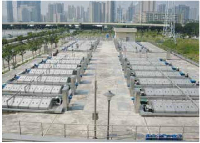
28 HUBER Disc Filter RoDisc® units with 24 discs each treating about 8.5 m<sup>3</sup> wastewater per second.
