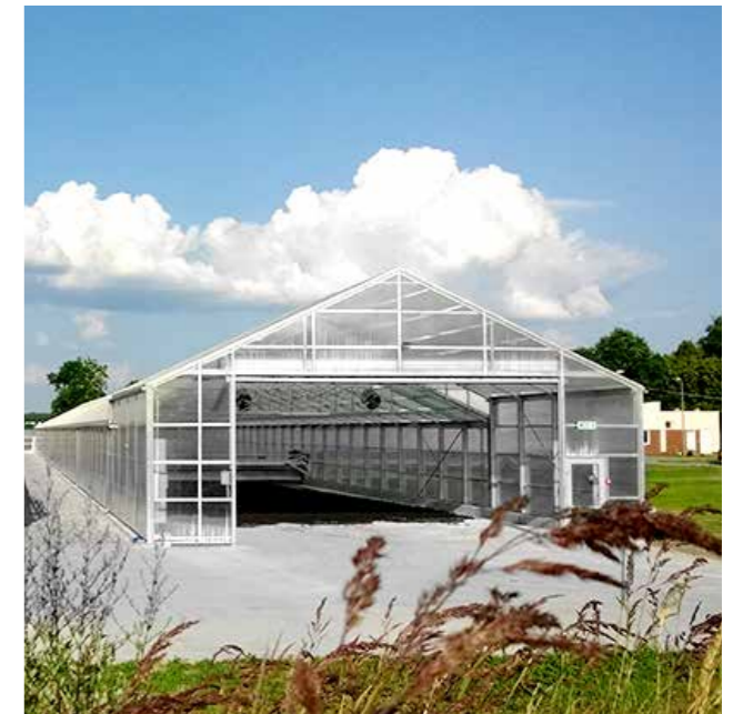
Dewatered sludge is transported in through gates.
